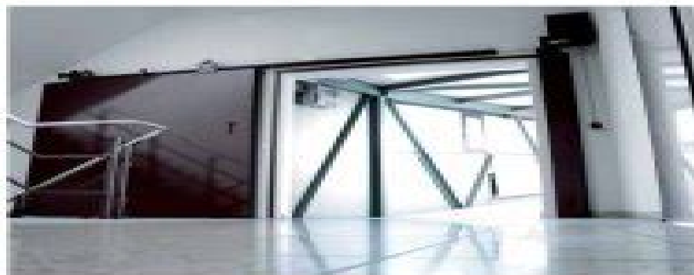
The Gilgen closing device BSV-FT is designed as a power-driven independent device of the manual free-ringed single sliding door leaf.
