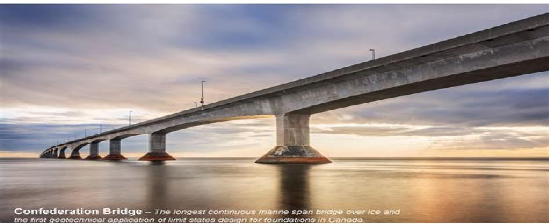
**Confederation Bridge** – The longest continuous marine span bridge over ice and the first geotechnical application of limit states design for foundations in Canada
